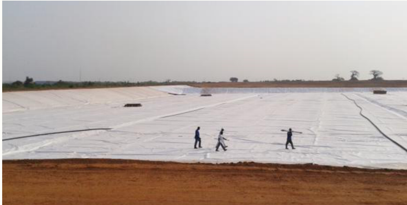
Placing of geotextyle fabrics
