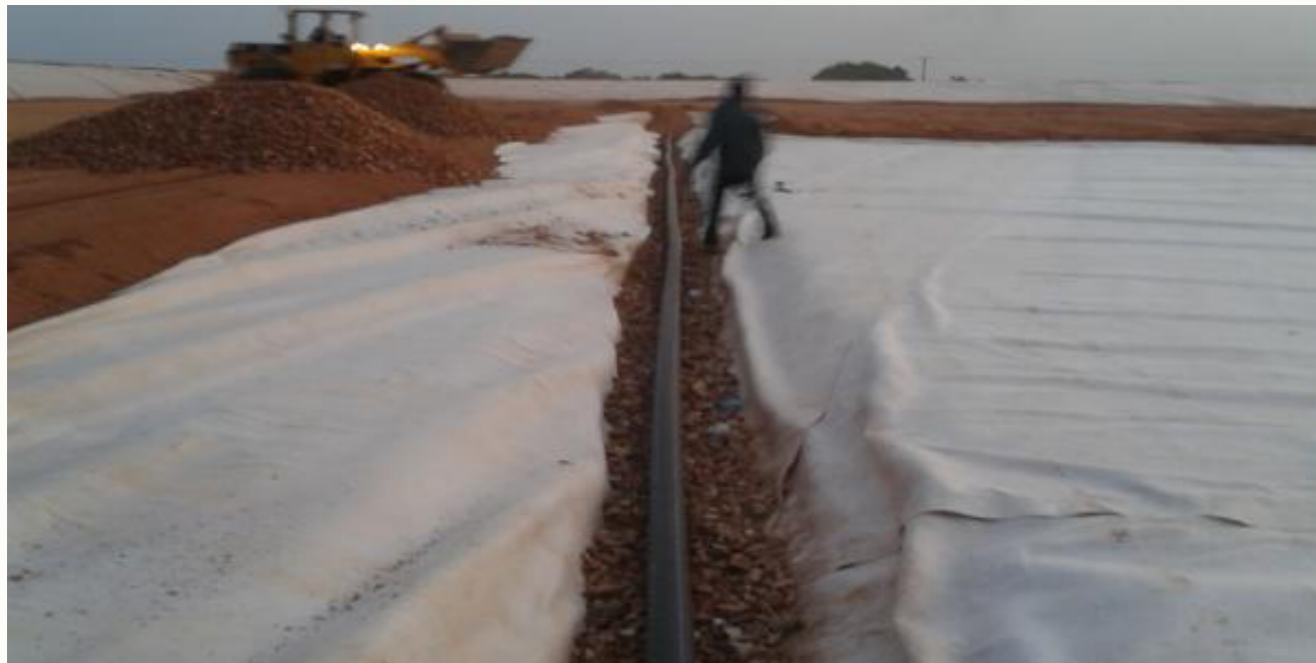
Lining of drainage channel
