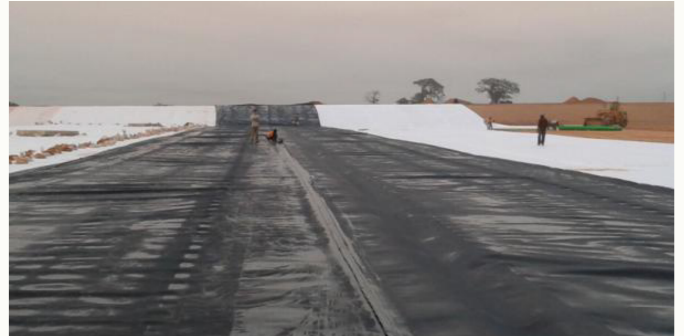
Welding of the geomembranes
