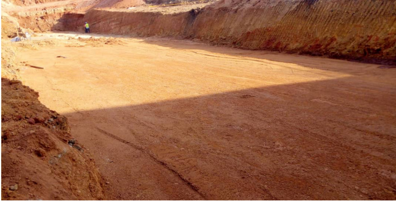
1. Excavation and ground preparation
