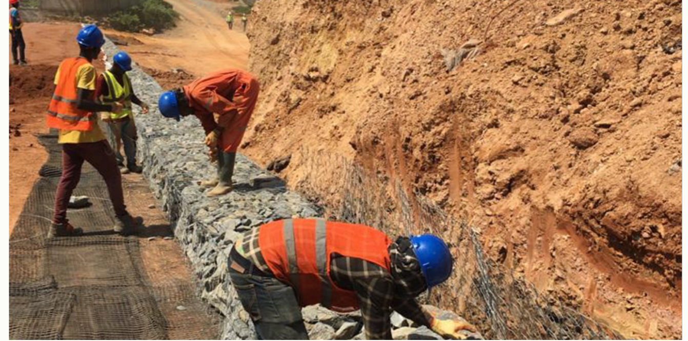
3. Filling the gabions with rocks
