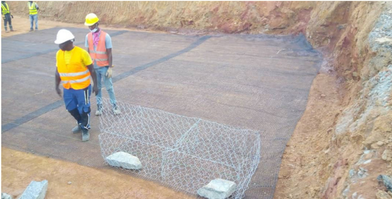
2. Placing gabions and laying geogrids
