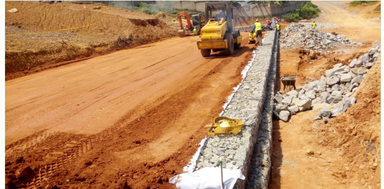
7. compaction - and back to step 1.
