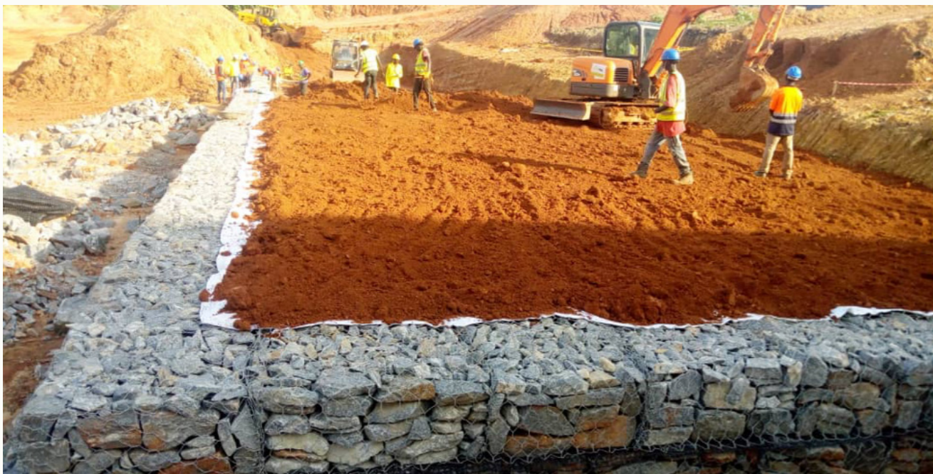
6. Second layer of 25 cm thick backfill material
