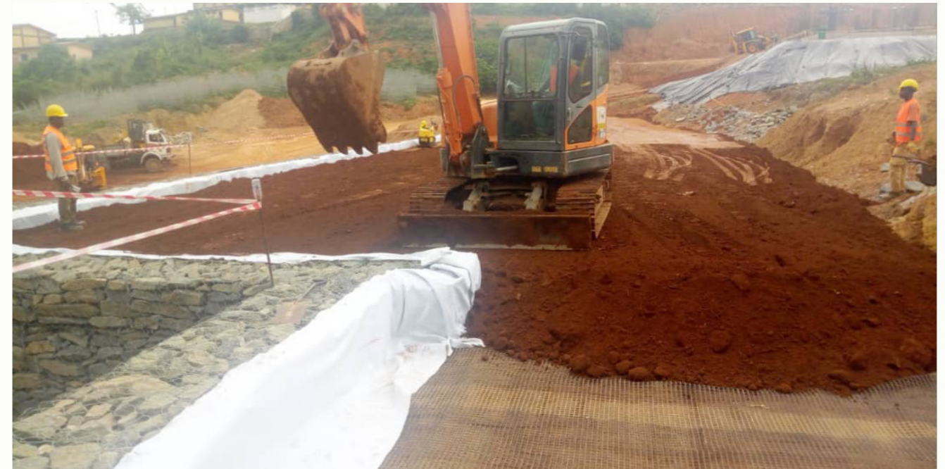
4. First layer of 25 cm thick backfill material
